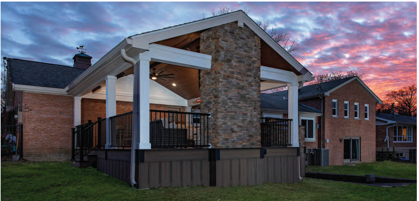
COZY OUTDOOR DECK , constructed by Jessica Hagan's company, All Decked Out, was built under an open gable roof next to an outdoor fireplace and custom outdoor kitchen. (Photo by LiVon Photography)
